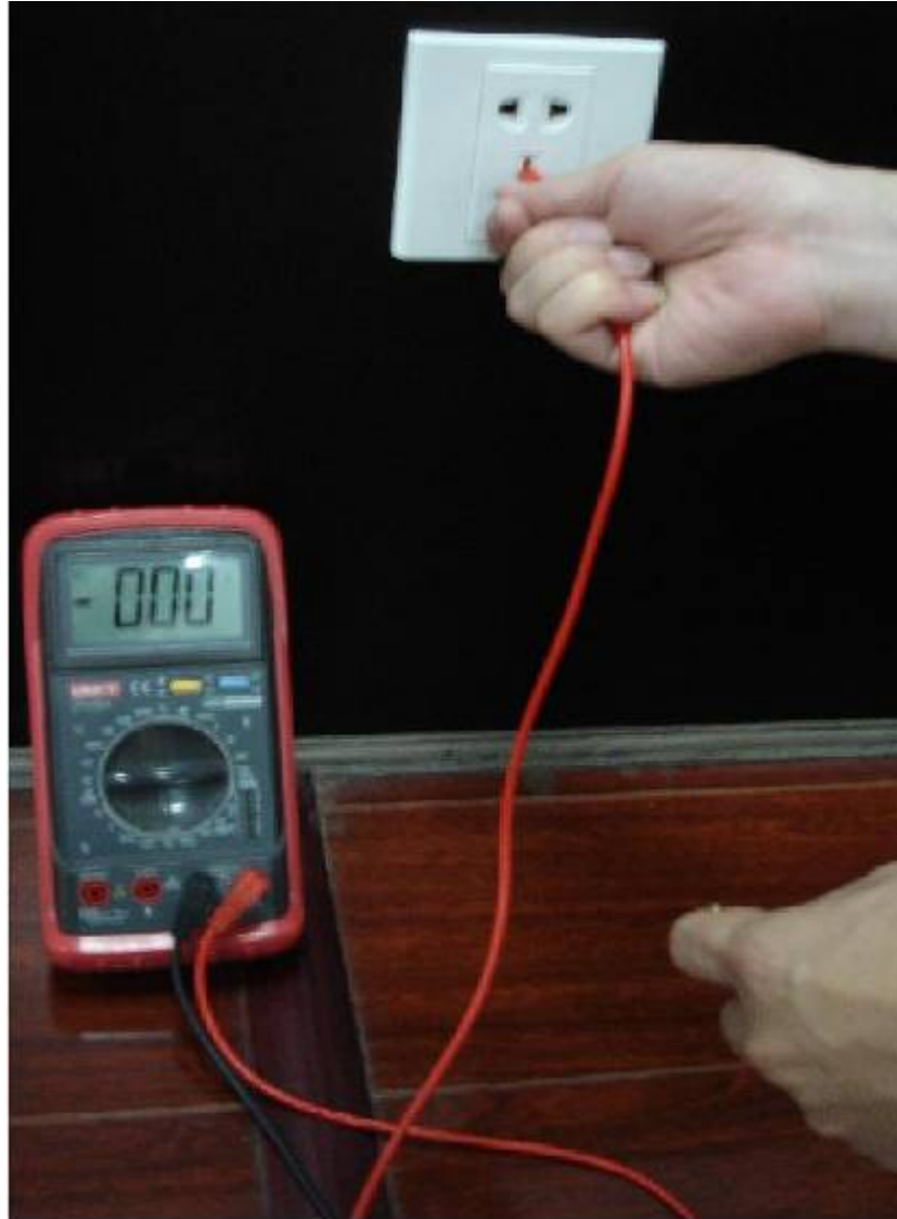
Appendix Figure 7-5 Check earth cable connection
