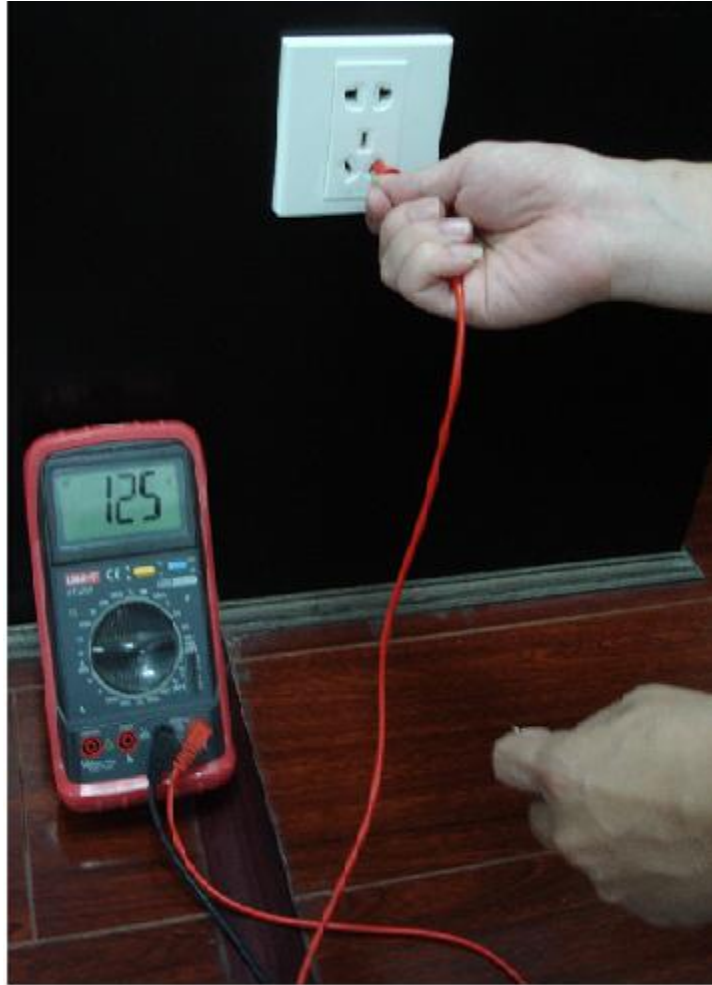
Appendix Figure 7-6 Check live cable connection
